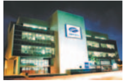
A $450 million investment in Banco del Progreso saved DR's financial sector from collapse
